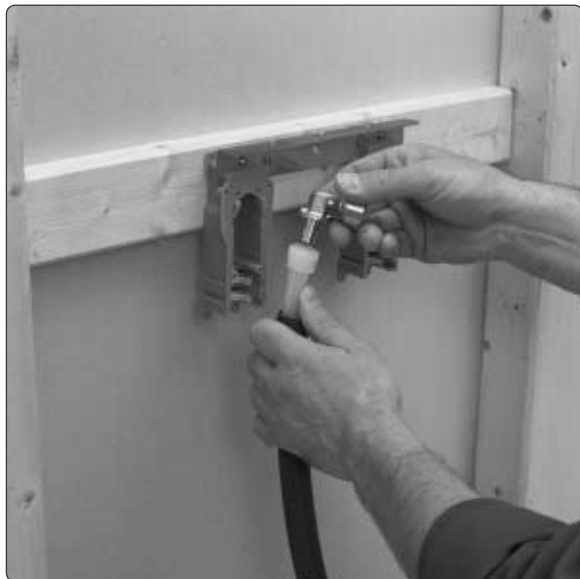
3. Montera Q&E-koppling.
